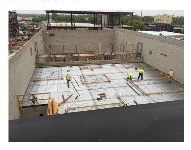
MECHANICAL MEZZANINE - A concrete floor will be poured above the Dance/Cheer Dressing Room for a mechanical equipment mezzanine.
