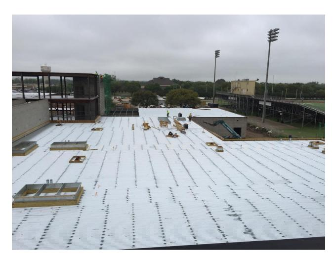
ATHLETICS – Steel roof decking is being installed over the boy's and girl's athletic spaces. A light-weight concrete roof deck will be poured over the steel roof deck in preparation for roofing dry-in.
